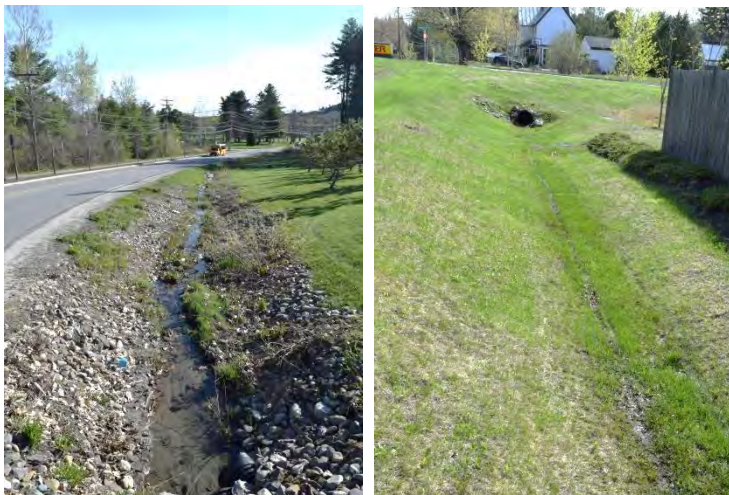
Figure 5. Examples of a drainage ditch and a grassy swale
