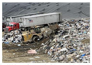
face before new waste was placed and compacted. Leaving thick lenses of compacted soil (or waste derived ADC) between the lifts of waste can be a contributing factor to leachate seeps and landfill gas compartmentalization.
