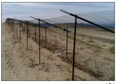
containing it within the fence. To be as effective as possible, this fencing needs to be periodically de-constructed and repositioned to the most effective locations. Dependent on on-site conditions and topography a series of temporary litter fences may be needed to collect and contain surface blown litter.
