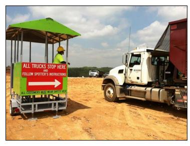
barriers. From the safety of the spotter station, the spotter can greet each customer, visually check loads, and provide verbal (face to face) direction. We recommend that the spotter stay in or is physically protected by the spotter station at all times, as this is the only way to truly protect them from hazards. When properly positioned, a spotter can adequately provide direction while viewing what is taking place at the tipping area.
