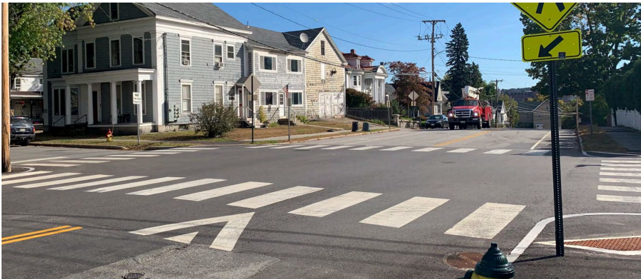
Auburn - Elm and High St. -Raised Intersection
