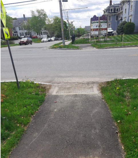
Bangor Main St Bump-Out – View From Sidewalk
