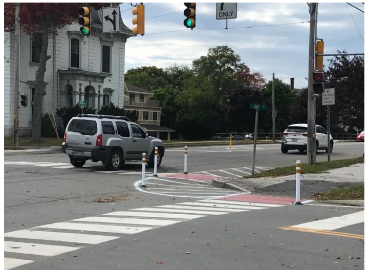
Bangor -State St - Radius Flattening and Crosswalk Bump-Outs
