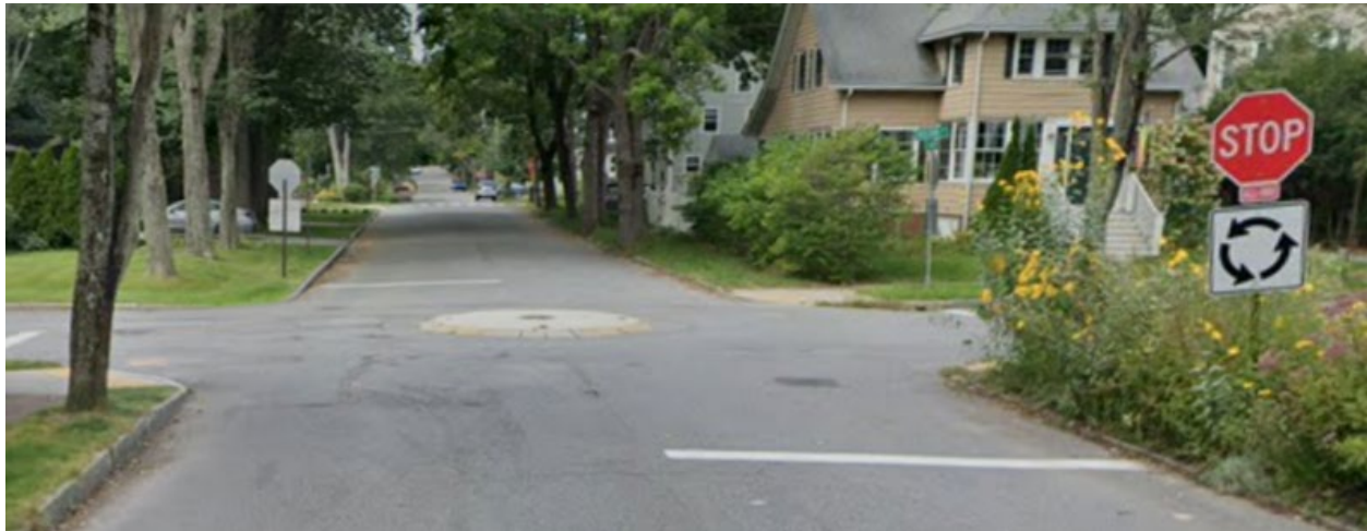
Portland - Neighborhood Roundabout - Elizabeth Rd and Bolton St
