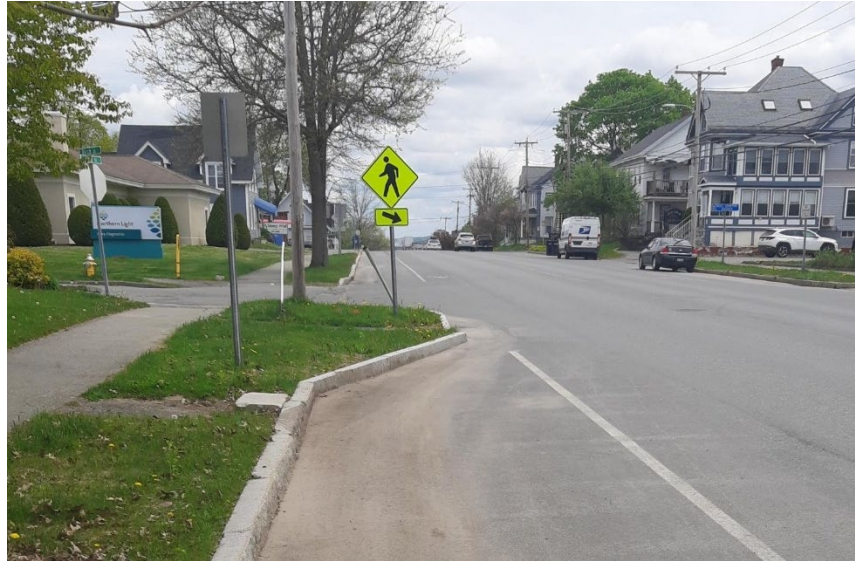
Bangor Main St Bump-Out-Shoulder View Showing Tapered Transition
