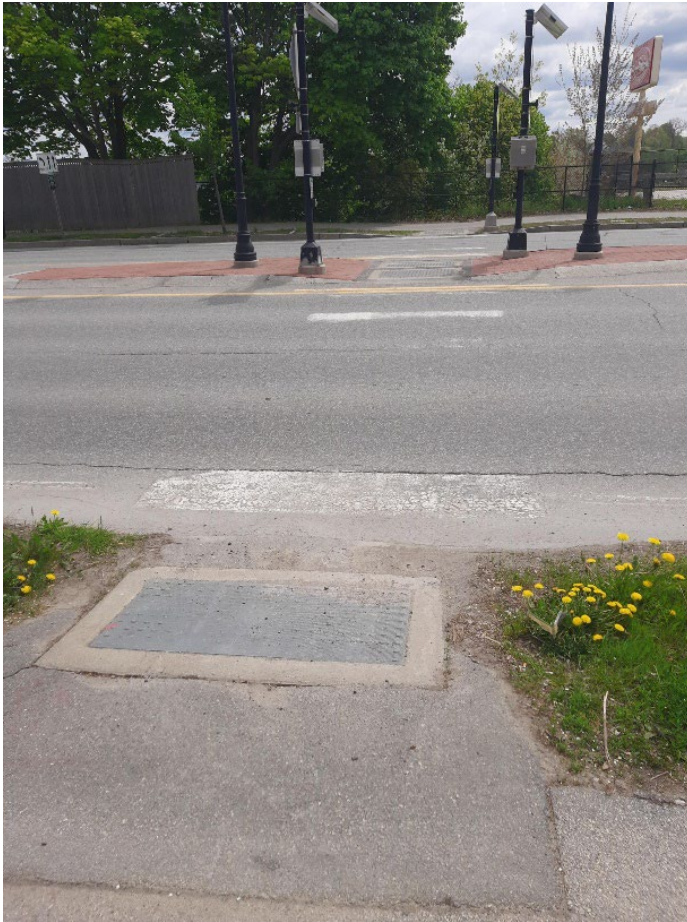
Bangor Main St Median Island Shown From Sidewalk
