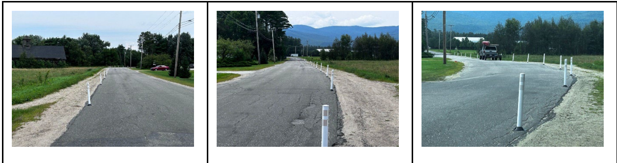
Figure 4—Visual barriers with vertical Flex Posts, Bethel, 2023
